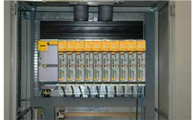
AC890 air ducting components make easy work of cabinet building when force ventilation is to be used. The exhaust duct, supplied in 1 meter sections, is mounted to the top of the AC890 heatsinks and includes a 190 CFM fan. This arrangement provides a very effective means of cooling by drawing air directly through the drives' heat sinks and out of the air outlets which can be flex-ducted out of the cabinet. See part numbers in table to right.
