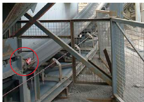
Lubrication of pillow block bearing on belt weigher
