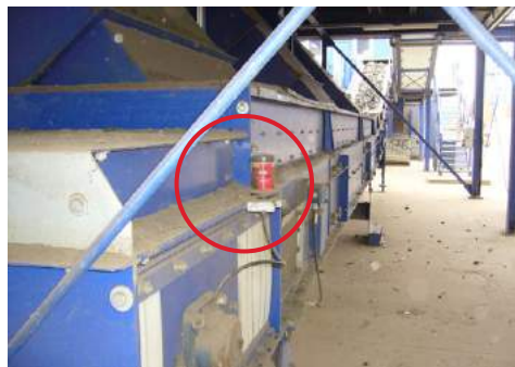
Lubrication of pillow block bearing on conveyor
