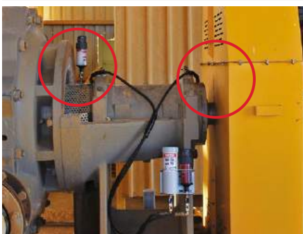
Lubrication of flange bearings and seals on pump
