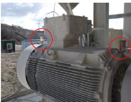
Lubrication of motor on a vibrating screen
