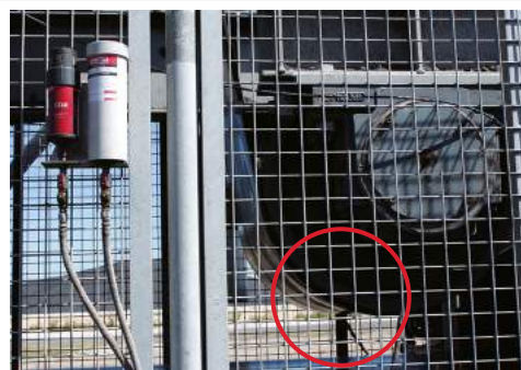
Lubrication of pillow block bearing on conveyor
