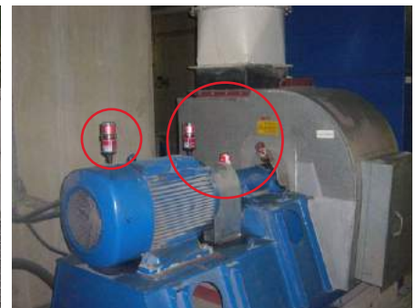
Lubrication of electric motor and shaft on secondary fan
