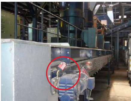
Lubrication of flange earing on conveyor
