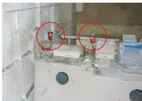
Lubrication of pillow block bearing on fan drive shaft
