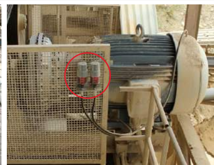
Remote lubrication of electric motor
