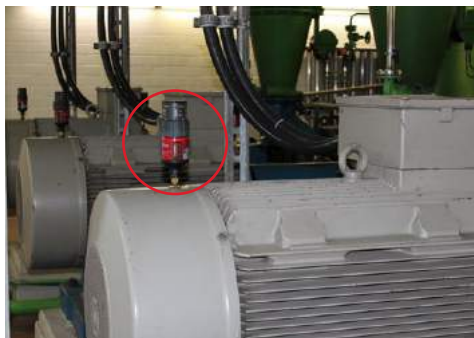
Electric motor bearing lubrication
