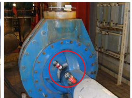
Lubrication of drive shaft on pump
