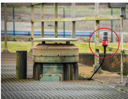
Lubrication of bearing at surface aerator
