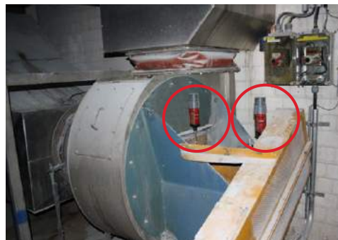
Lubrication of pillow block bearing on a ventilation system
