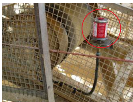
Lubrication of pillow block bearing on conveyor
