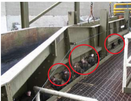
Bearing lubrication at the tree sorting system
