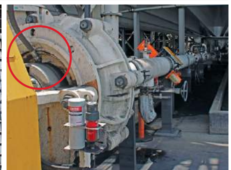
Pump bearing lubrication
