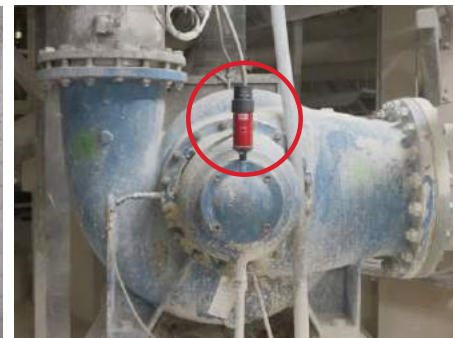
Pump bearing lubrication
