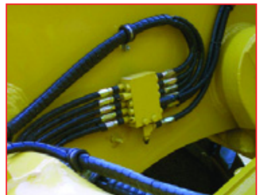
Lincoln system houses have experience to ensure installations are clean and neat
