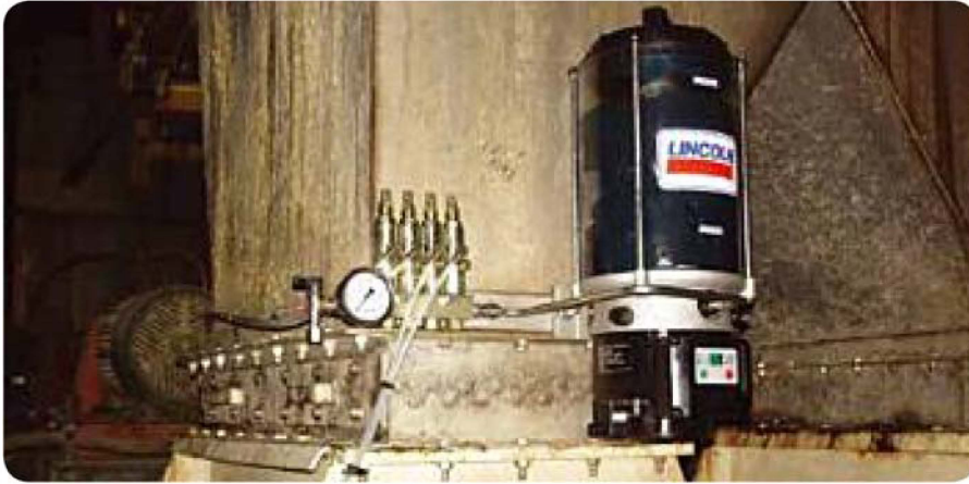
This Centra-Matic automatic electric pump and injectors are lubricating bearings in a very abrasive and dusty environment.
