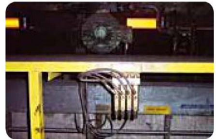
These SL-V injectors operate in a harsh steel mill environment that includes high heat and abrasive contamination. Purging the bearings, replacing the grease film frequently and increased safety are key benefits of this system.
