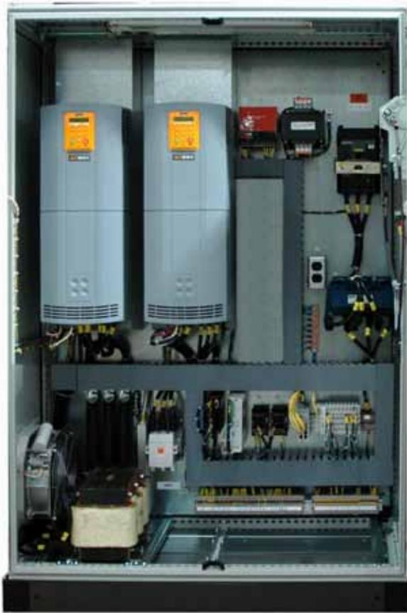
Illustration shows typical panel including AC690+ with AFE and additional system components.
